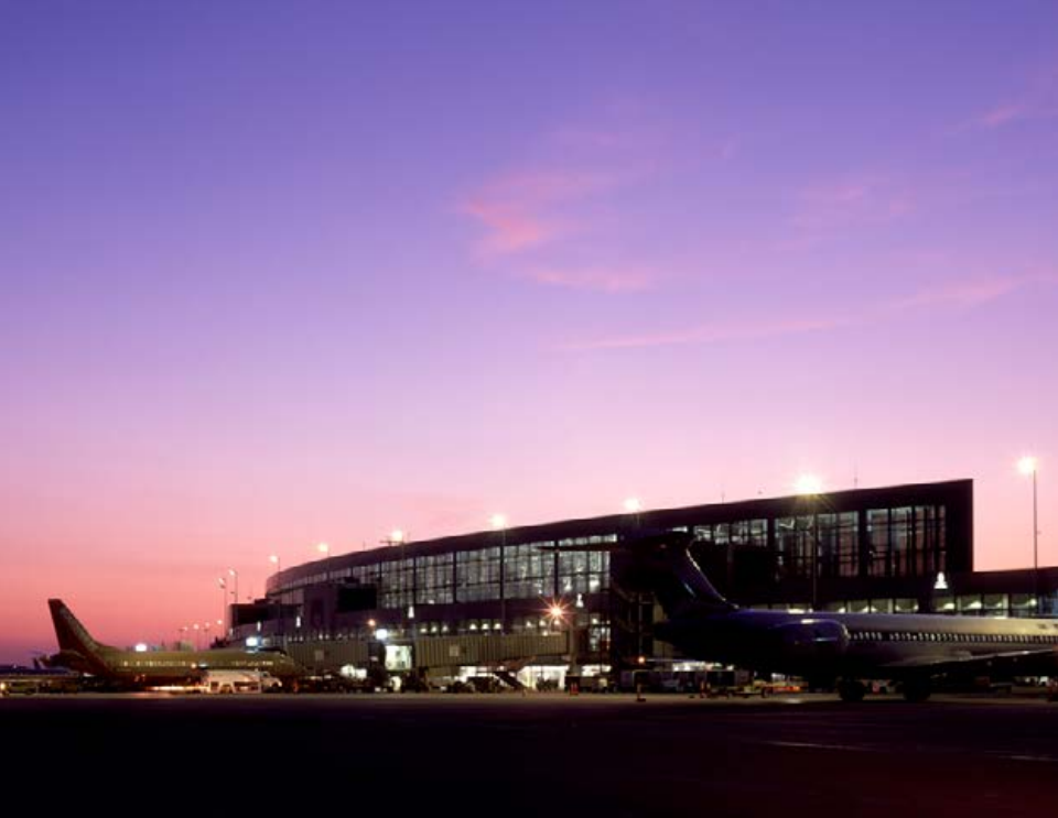
Photo by Austin Bergstrom International Airport
