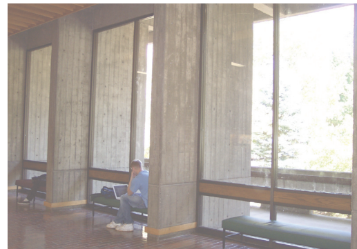
McKenzie interior showing roughcast concrete.
