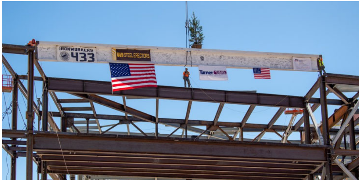
Beam Hoisting Ceremony of Las Vegas Convention Center Expansion
