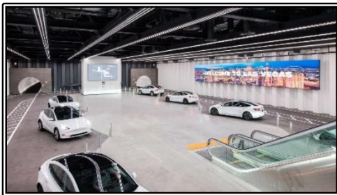
Las Vegas Loop Central Station
