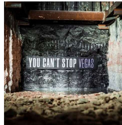
LVCC Loop Tunnel During Final Construction
