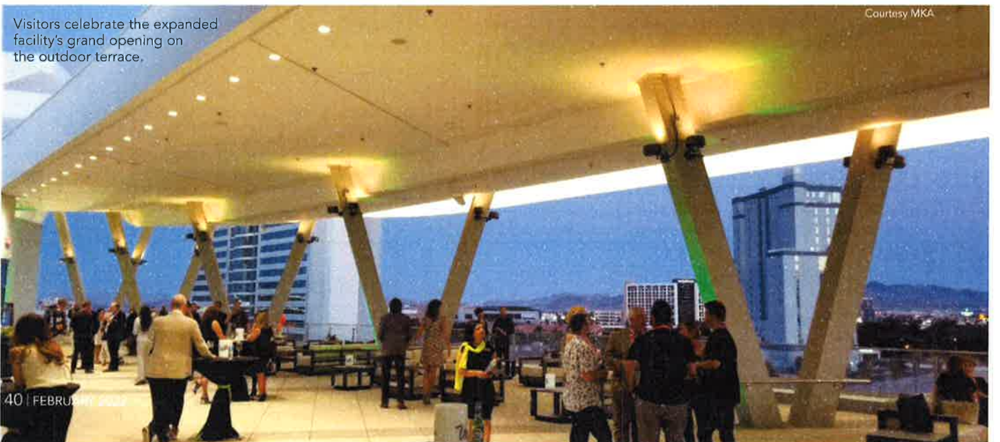
The long cantilevers allow the ribbon roof to "float" above the outdoor terrace space and provide shade and comfort for visitors.
