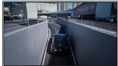
Las Vegas Loop Tunnel Exit
