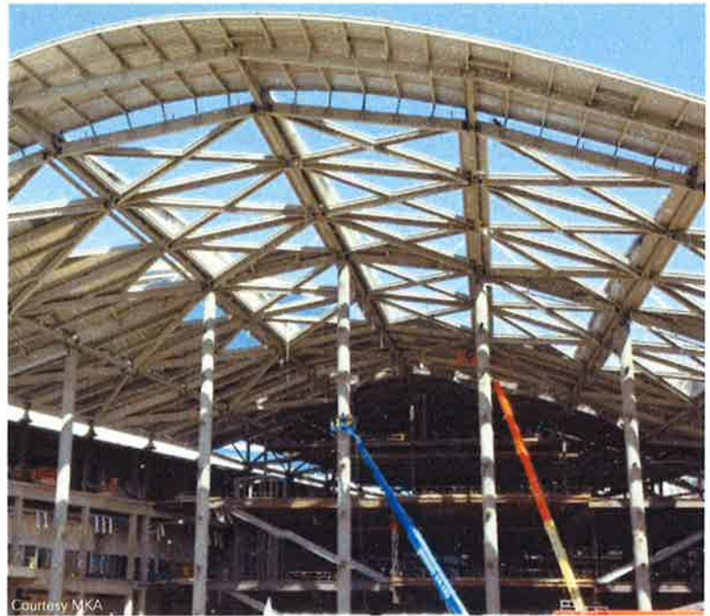
above: The lobby's “snow cone” roof cantilevers 125 ft to the south of the entry wall.
