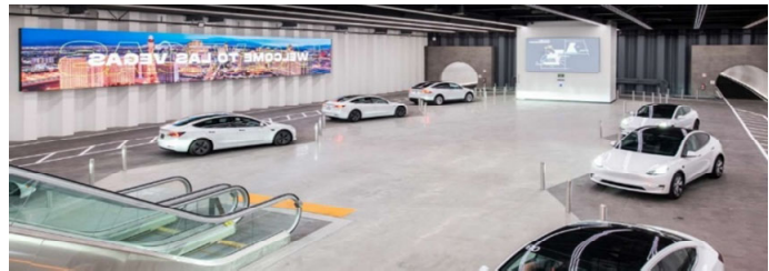
Las Vegas Loop Central Station
