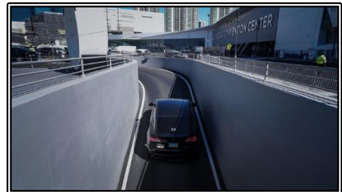
Las Vegas Loop Tunnel Exit
