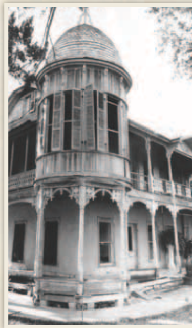
H.D. Gruene's home, now Gruene Mansion Inn, built 1872.
